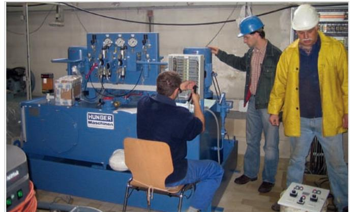
Installation of cylinders, hydraulic power unit and execution of the piping at the hydro electric power station Wallstadt, Germany
